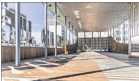
The rooftop at the Contemporary Austin's Jones Center on Congress Avenue features a new canopy and weatherproof curtains. RICARDO B. BRAZZELLI/AMERICAN-STATESMAN
